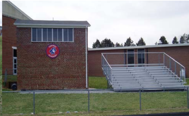
Concession Stand and Press Box with Restrooms located near Seating
